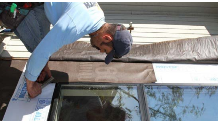
Photo below: Careful attention to proper lapping of building papers and flashing at window replacement project
