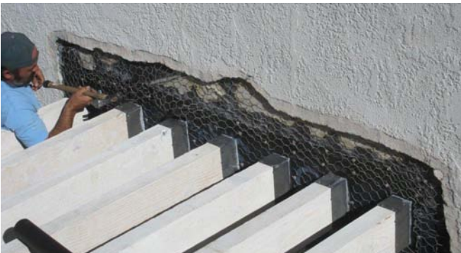
Photo below: Careful attention to proper lapping of building papers and flashing at window replacement project
