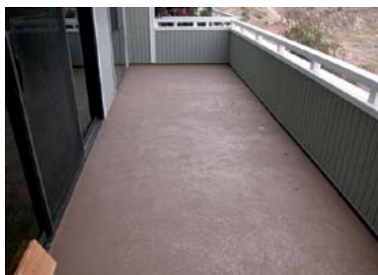
Balcony with a solid waterproofed finished floor
