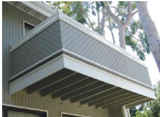
Reconstructed cantilevered balcony
