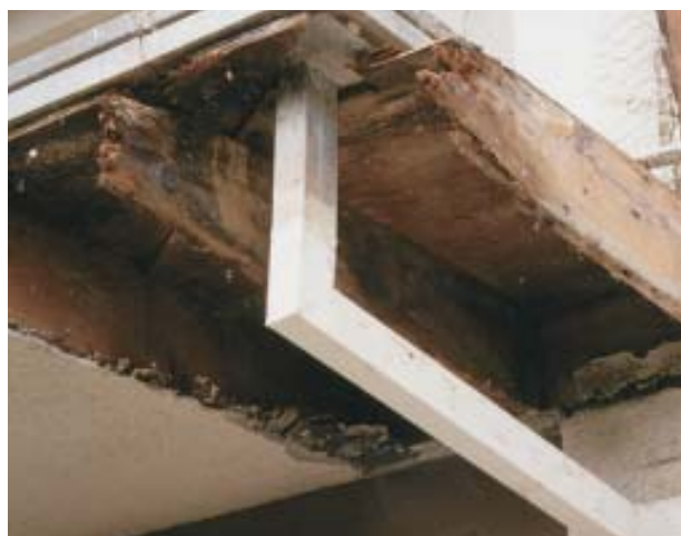
Figure 2. Improperly flashed scuppers (left) and floor drains (right) often allow water into the framing, leading to hidden rot.
