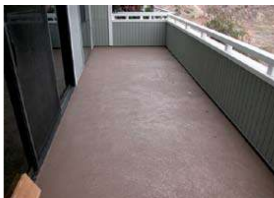
Balcony with a solid waterproofed finished floor
