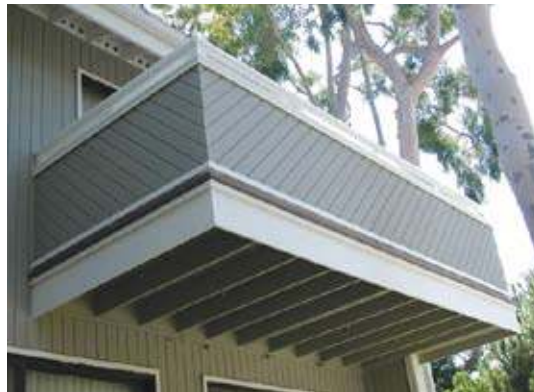
Reconstructed cantilevered balcony
