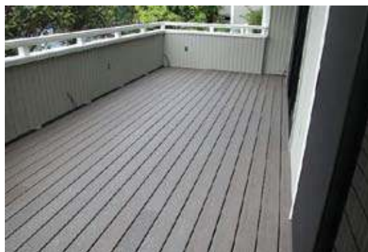
Balcony with a gapped decking finished floor
