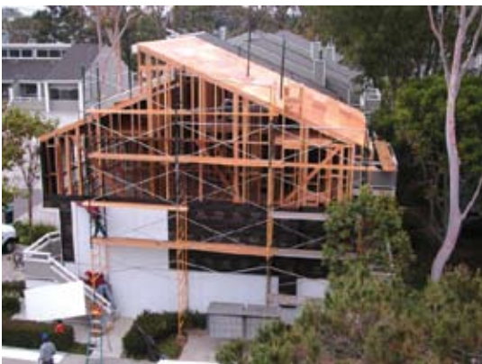
New siding installation on townhome damaged by fire
