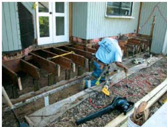
Replacement of decayed beam supporting entry balcony to condo
