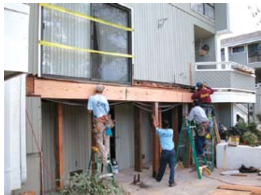
Reconstruction of decayed lower rear balcony
