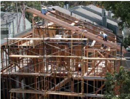
New roof framing being installed on townhome damaged by fire
