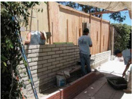
New masonry wall construction after automobile damaged condominium association perimeter wall
