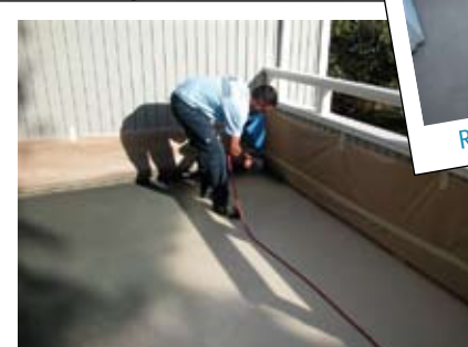
Application or waterproofing texture on condominium balcony
