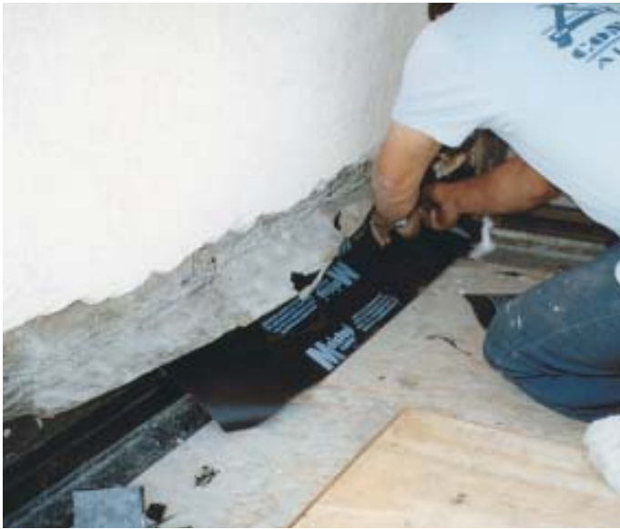
Figure 5. Flexible membrane flashing, tucked behind existing building paper and overlapping a sheet-metal skirt flashing, provides positive wall drainage onto the new balcony surface.
